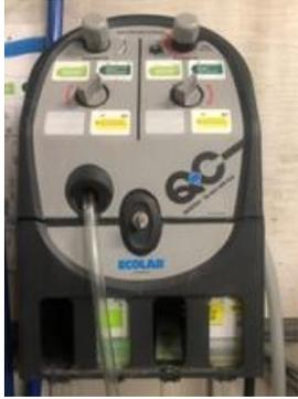
The installation of a pre-plumbed chemical proportioning system to help to assure the proper level of cleaning agent is used at the stations was also installed at both stations. This system will also help reduce the excess product usage from an unregulated system. Plus, all the products are from a local business.
